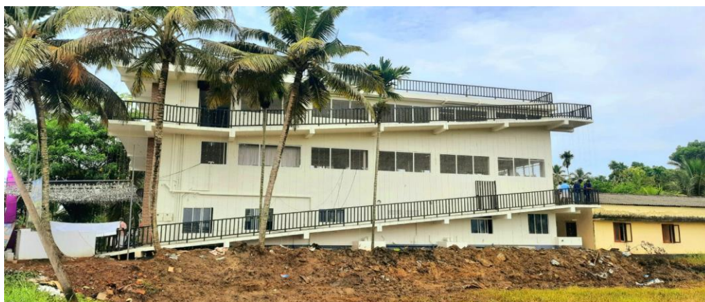
Elevated And Community Cattle Shed at Chempumpuram Dairy Co-Operative Society (Ltd No. 156(D) APCOS) - Inaugurated On 12.05.2022
